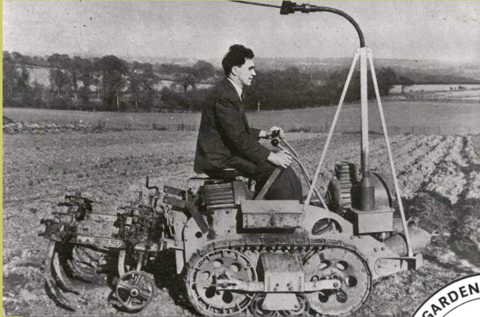
Prototype electric Ransomes MG crawler. Photo believed to be taken at Ransomes Nacton test ground.
